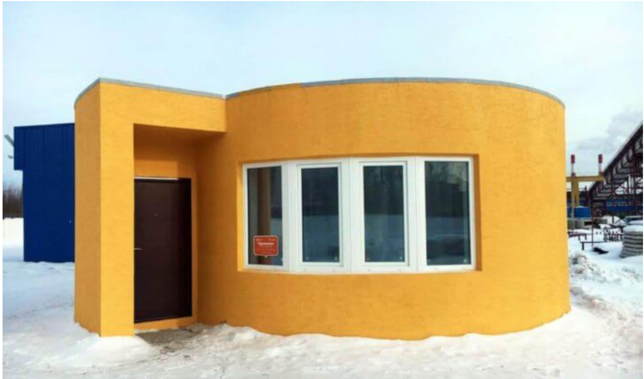
Illustration: house claimed to have been built in 24 hours with 3dprinting
